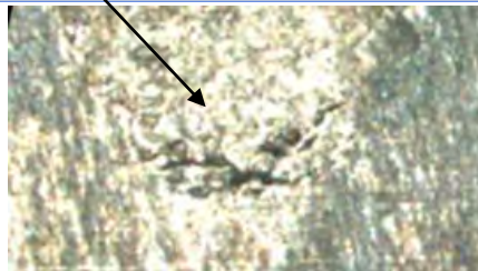
75-mil Crack Cluster (Maximum Crack Length 50 mils)
